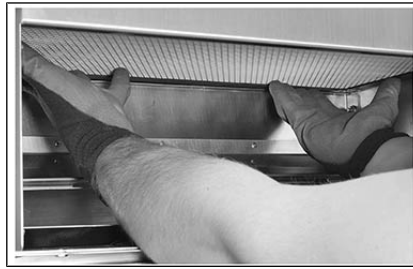
Image: Replacing air filters
